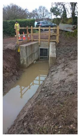
In Snakes Wood, two 600mm penstock sluices have been installed above an existing culvert. In recent years, considerable volumes of water have flooded into the Canal at Atherton way in Tiverton. This overflow into the canal has been formalised with open grilles on manhole covers, surrounded by bunds in order to ensure that floodwater is directed into the canal rather than flooding
